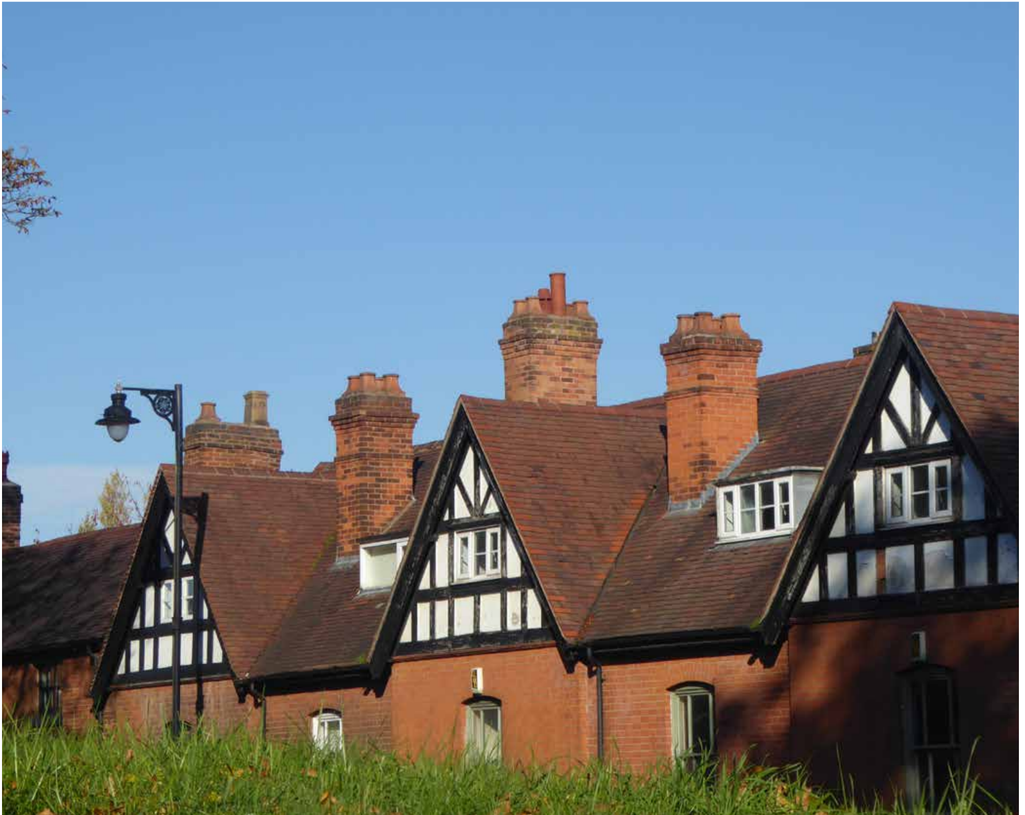
Distinguishable Chimneys & Rooftops, Sutton Coldfield.
