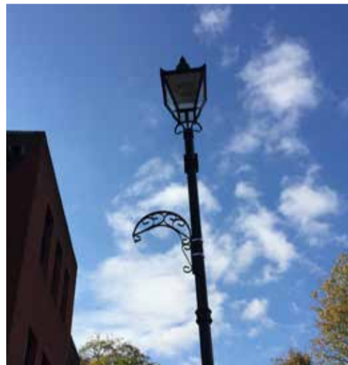
Ornamental street lighting.
