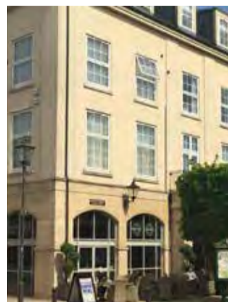
Large glazed commercial frontages support vertical emphasis of the architecture.
