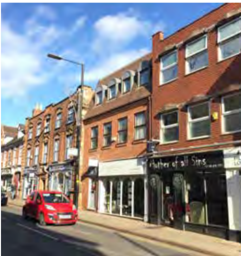
Continuous building lines. Later infill developments have respected this approach.
