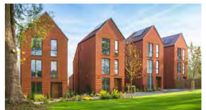
Narrow, regularly spaced detached plots can provide an alternative method of stepping down steeper gradients without the need for significant cut and fill or retaining structures.
