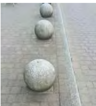
Stone balls define the pavement/ road edge. Also assists parking controls and security for the retail units.
