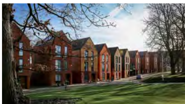
Narrow, regularly spaced detached plots can provide an alternative method of stepping down steeper gradients without the need for significant cut and fill or retaining structures.
