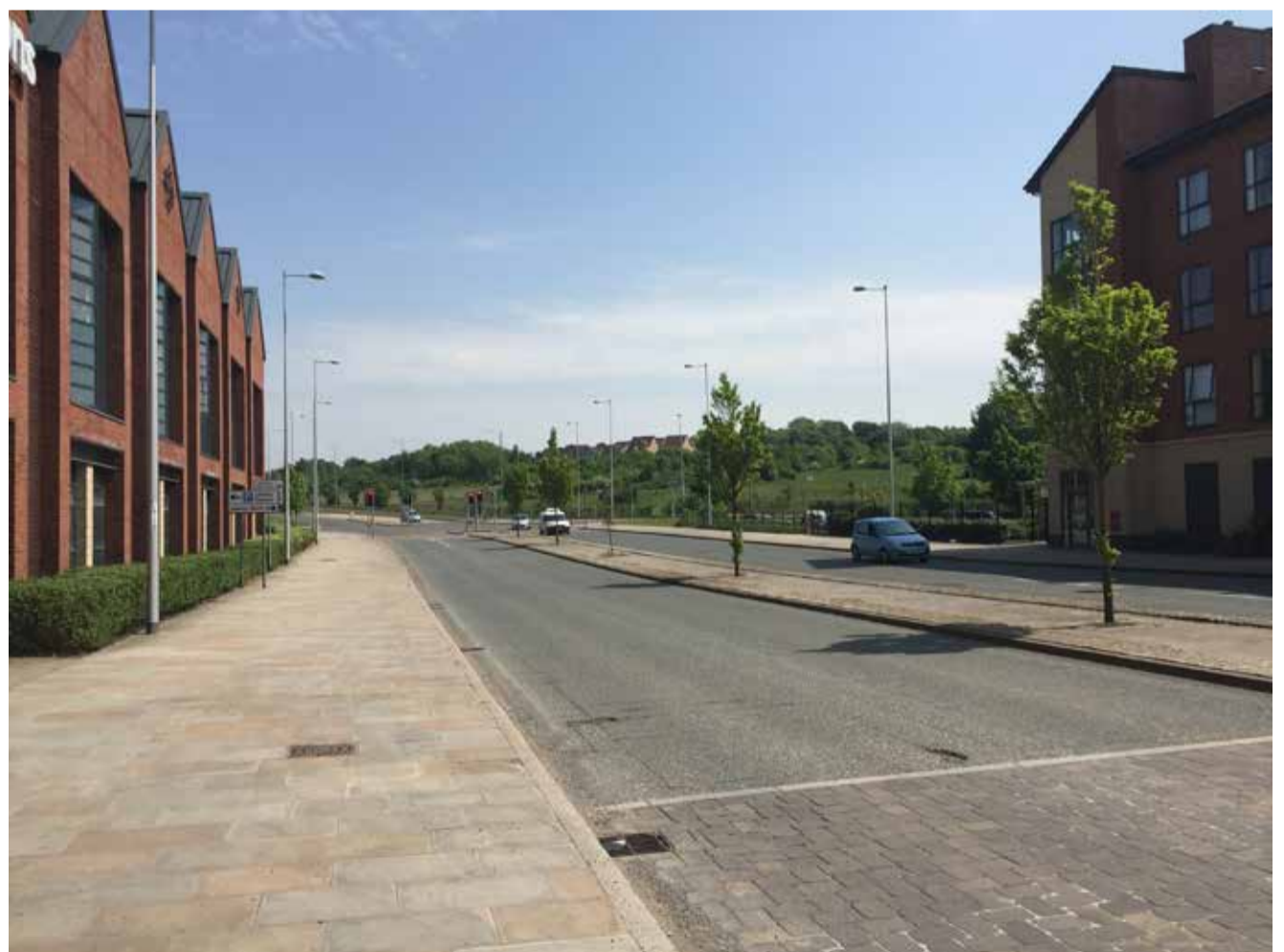
B5072 - The main connecting road from the A5223 towards Telford.
