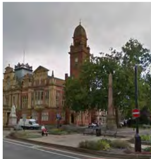
Landmark clock tower demarcating civic use.
