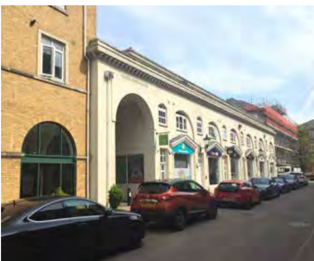
Archways evident throughout the architecture. Change in height also helps to reduce the sense of enclosure felt in other parts of Main Street.
