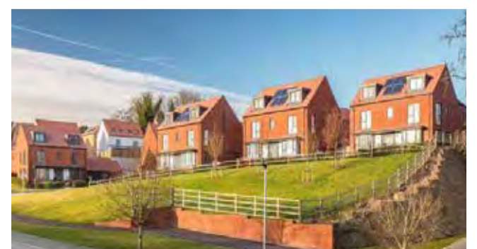
Areas of incidental space do occur on topographically challenged sites, particular at corners. These instances should consider landscape treatments carefully to enhance character and improve the setting of built-form.
